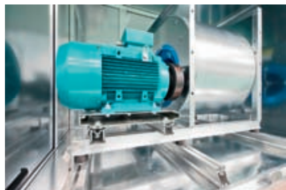
Figure 6: Close-up of fan-motor assembly (offset motor)
