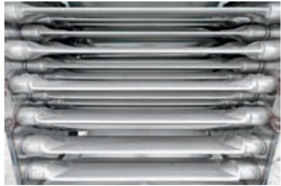
Figure 12: Gas heater exchanger
