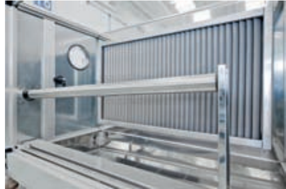
Figure 5: Isothermal humidifier steam pipe and droplet eliminator
