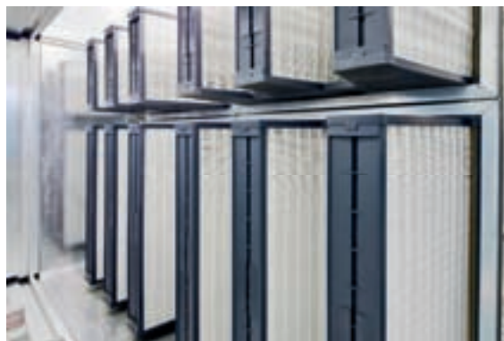
Figure 2: Rigid bag filters
